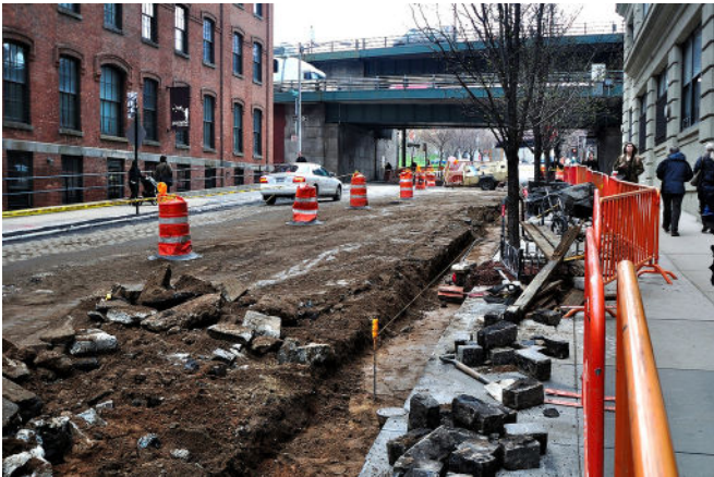
Construction on Washington Street, New York, NY
