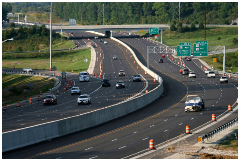
Interstate 69 Construction Project, Bloomington, IN
