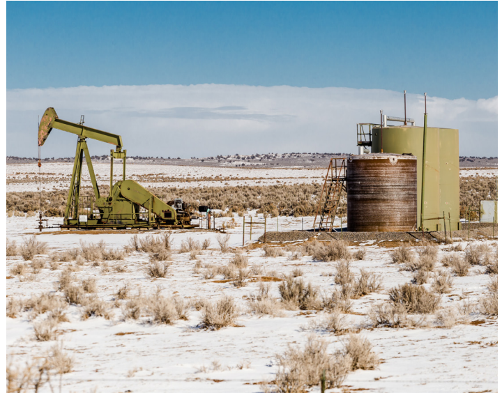
Lonely oil pump in the middle of a snow covered desert landscape on clear day in rural New Mexico by Richard, Adobe Stock
