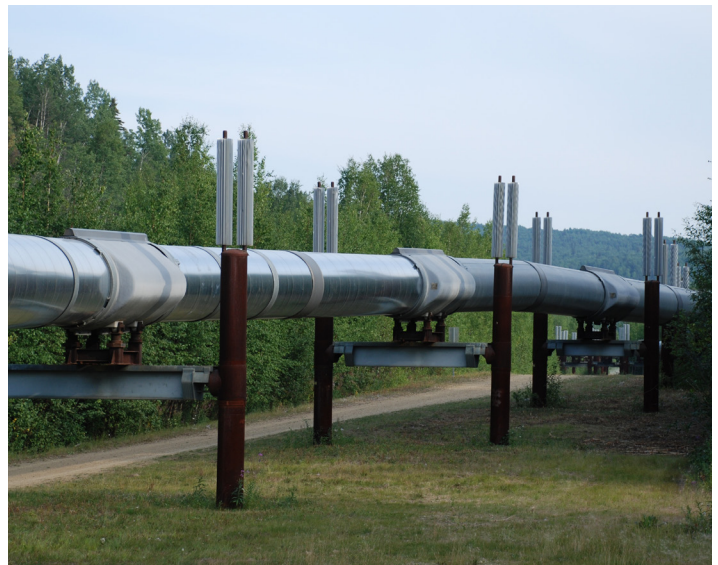
Oil Pipeline in Alaska U.S. Geological Survey Photo, Public Domain
