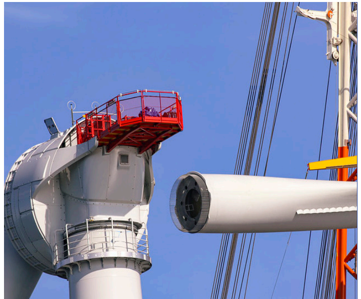
“Offshore_Turbine_Install_17” by Bureau of Ocean Energy Management , CC BY-SA 2.0
