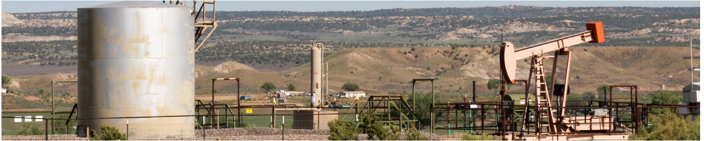
Oil Pumping Site in New Mexico by Kara Grubis
