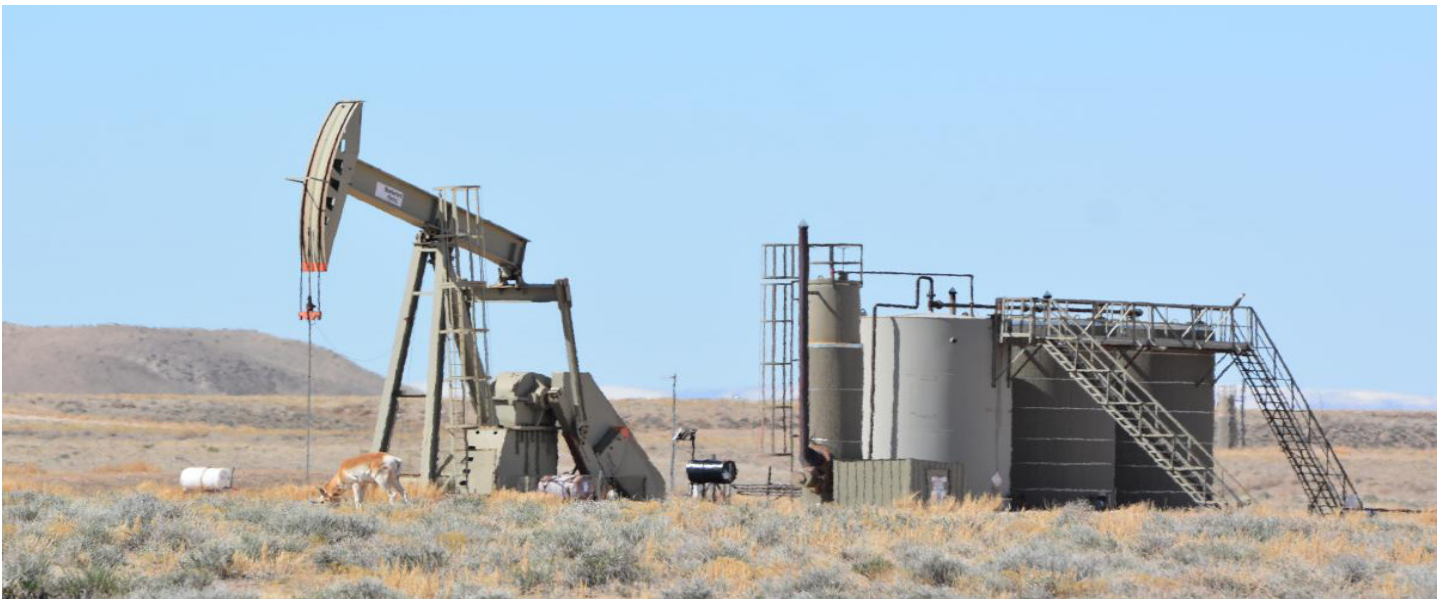
Oil pumpjack in Vernal, Utah area. BLM Photo
