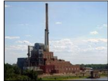
DOE's Proposed Plant to be retrofitted for FutureGen 2.0
