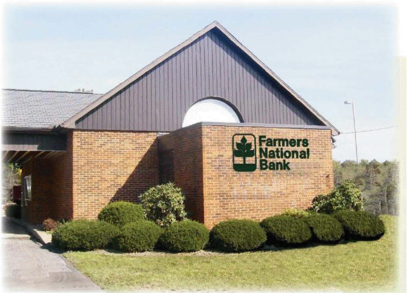
The new banking office located in Grove City, Pennsylvania.
